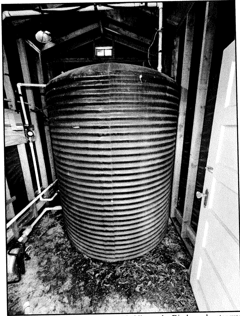
Photo 3: View of "Hansen Well" shed and holding tank. Discharged water was initially pumped to fill this tank before transferring to the sewer cleanout.
