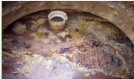
Clean grease interceptors routinely
